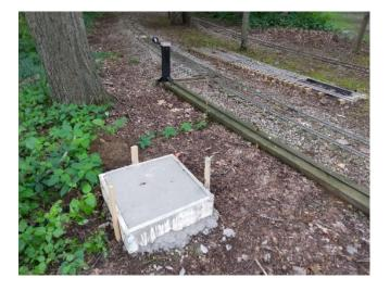
Approaching Soo Junction bases are in place for signals. The triangular aluminum frames behind the barn will make nice cantilever arms.
