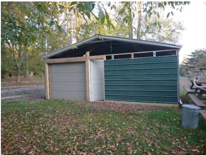
A couple weeks later the barn is almost ready for winter. This will give us more space to store equipment and give a permanent location for track panel and switch building.
