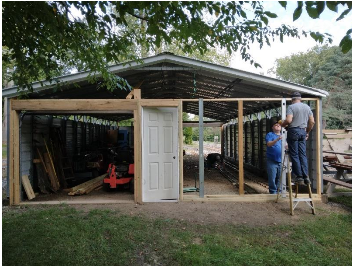
Tom Stick and Mike Schmitzer framing in the end of the barn.
