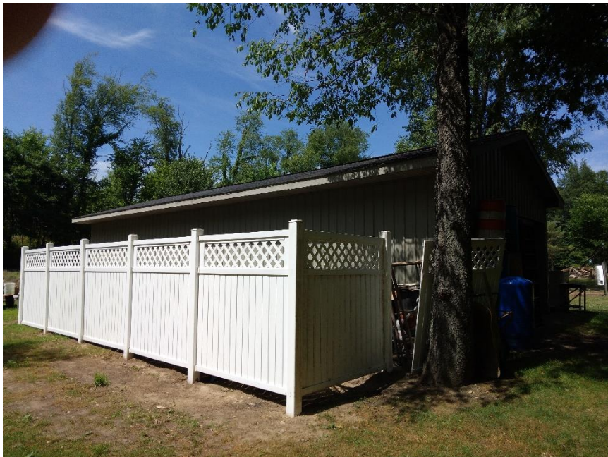
The fence Tom Stuck donated to hide the materials behind the barn. Like all railroads we have a variety of materials stored but our pile was becoming a bit unsightly.
