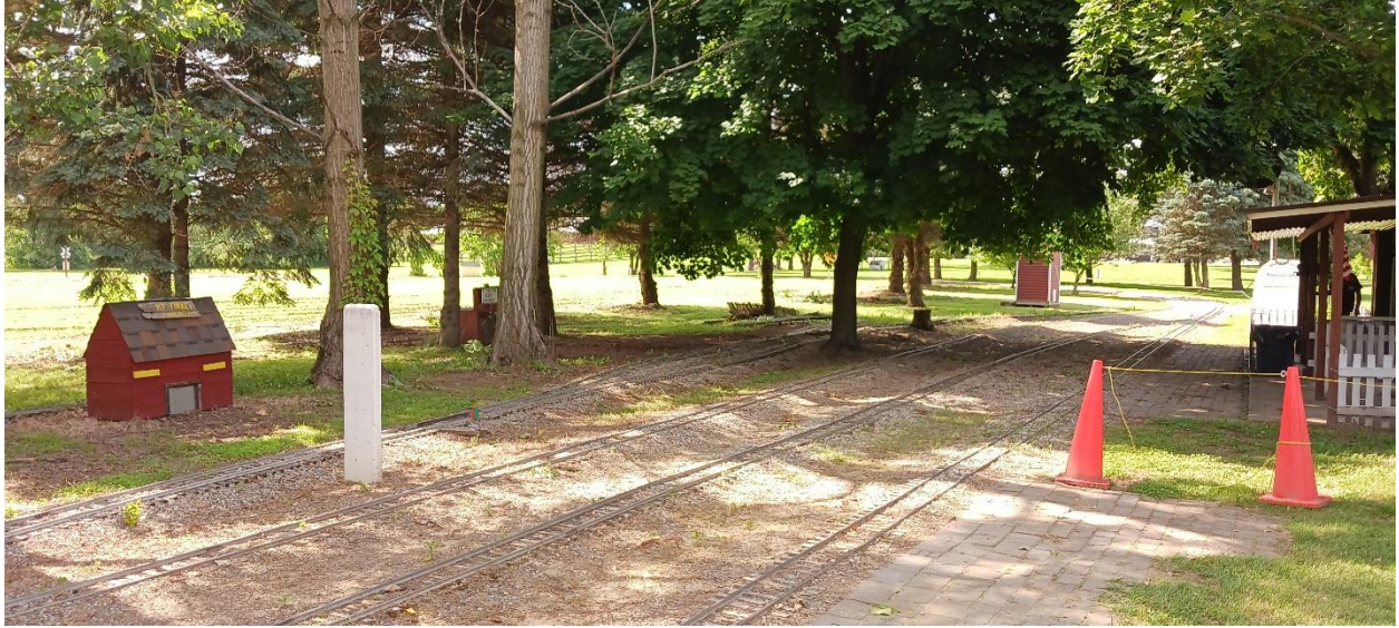
June 12 th was a slow day so the M of W forces went to work trimming trees.
