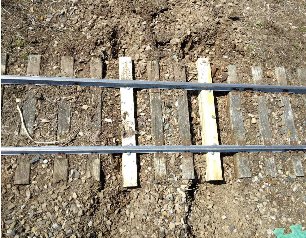
The Never Ending Story railroad edition, tie replacement.
